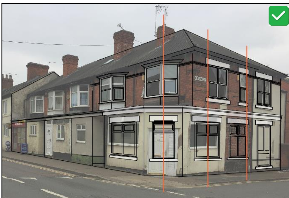
Preferred arrangement. Lower floor windows are aligned with the upper floor and window heads are replicated.
